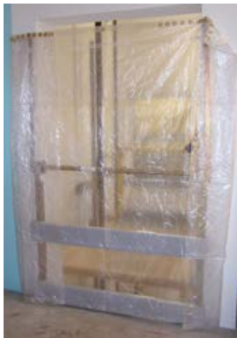
Variant 2: Extensive lift shaft entrance protection
