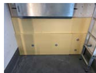
Hard foam board placed
