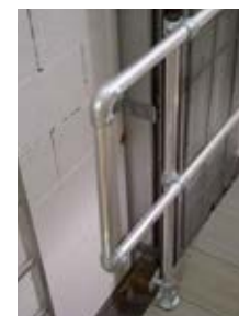
Closed run of the guard rail to avoid accidents
