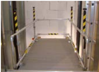
Car guard rail retracted
