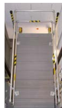
Closed run of the guard rail to avoid accidents
