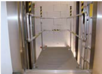
Car guard rail extracted
