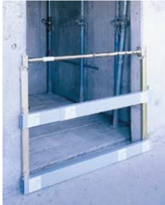
Variant 1: Partial lift shaft entrance protection
