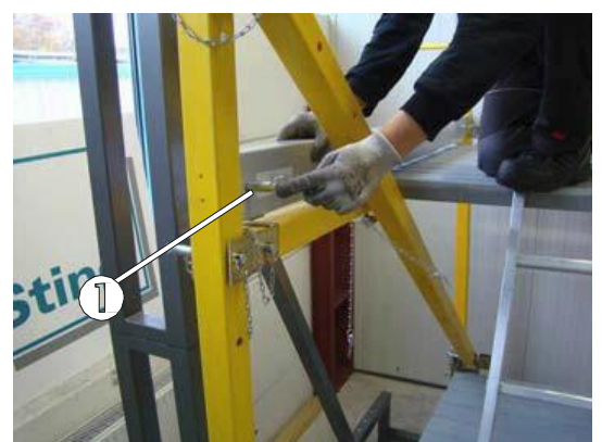
Fig. 91: Securing the foot rail
