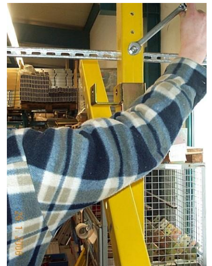
Fig. 41: Inserting the washer to distribute the force
