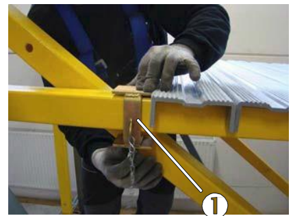
Fig. 82: Tube clamps to prevent the floor panels from slipping
