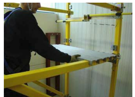
Fig. 77: Laying the upper floor panels
