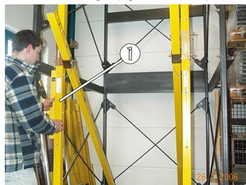
Fig. 38: Aligning the front vertical side of the triangle (right-hand side)
