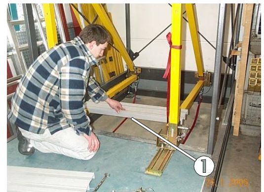
Fig. 16: Laying the first standard panel
