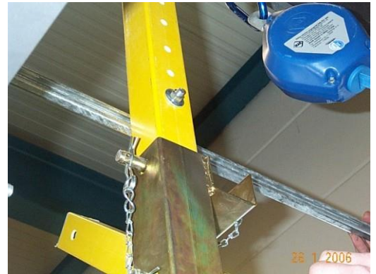
Fig. 40: Attaching the upper cross beam
