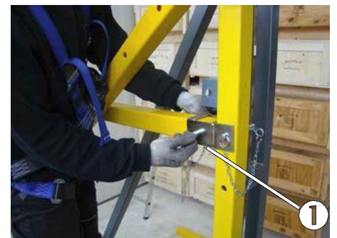
Fig. 64: Fixing the panel bars
