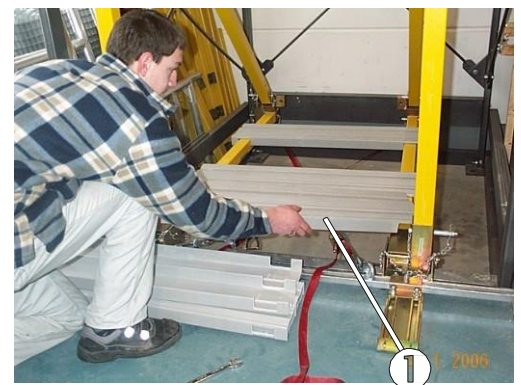
Fig. 32: Laying the other floor panels
