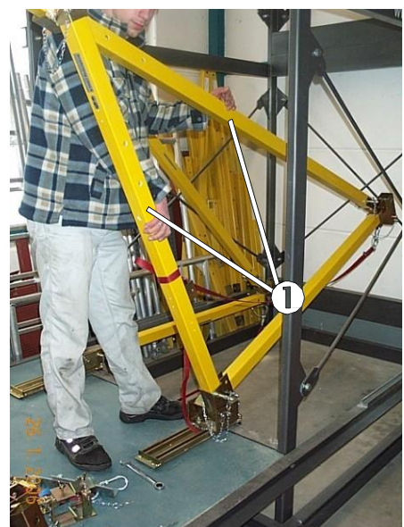
Fig. 14: Tipping the triangle element to the intel
