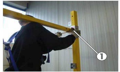
Fig. 54: Location points of upper horizontal bars
