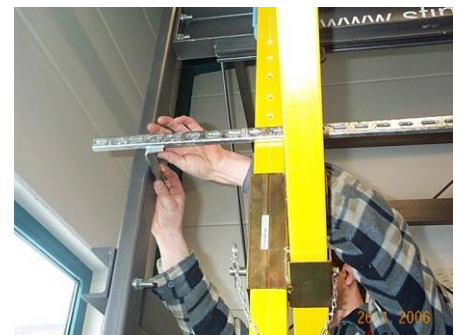
Fig. 43: Attaching the second L angle
