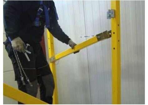
Fig. 51: Mounting the rear long bar
