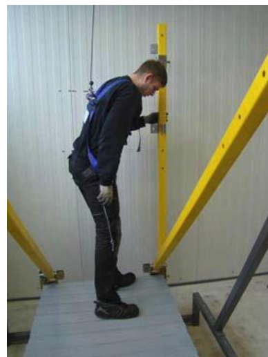
Fig. 45: Inserting the rear vertical rail stanchion
