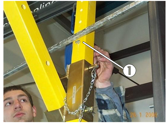
Fig. 40: Attaching the upper cross beam
