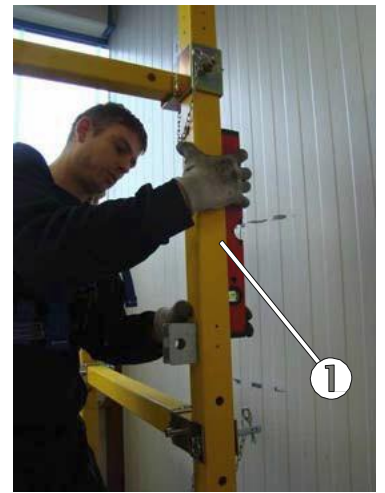
Fig. 59: Alignment of the rear vertical rail stanchions
