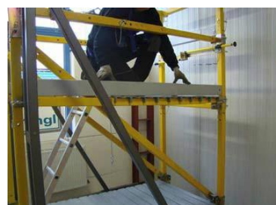
Fig. 91: Securing the foot rail
