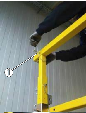
Fig. 86: The outer tube of the handrail is placed on top of the rear vertical rail stanchion
