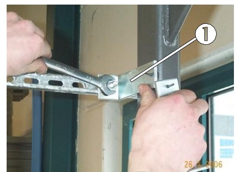
Fig. 44: L angle for the upper cross beam
