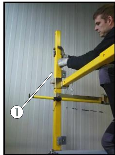
Fig. 73: Securing the upper vertical rail stanchion
