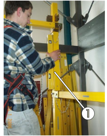
Fig. 59: Alignment of the rear vertical rail stanchions
