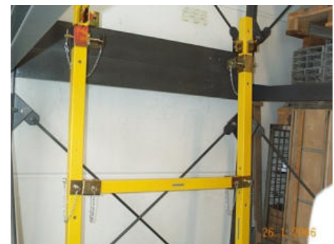
Fig. 52: Locking pins for securing the handrail
