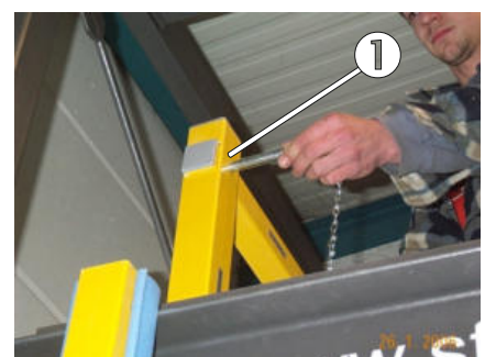
Fig. 95: The inner tube of the hand rail is inserted into the front vertical rail stanchion and secured with a locking pin
