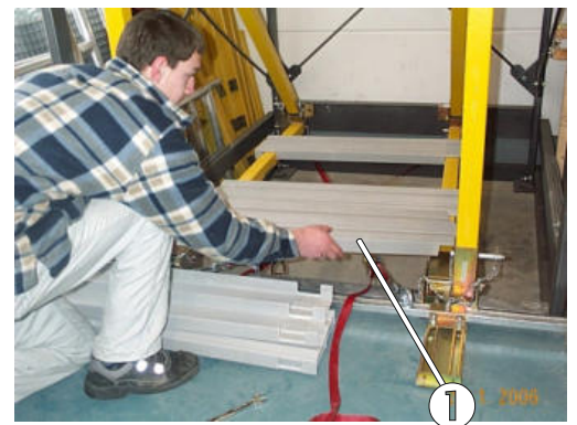
Fig. 32: Laying the other floor panels
