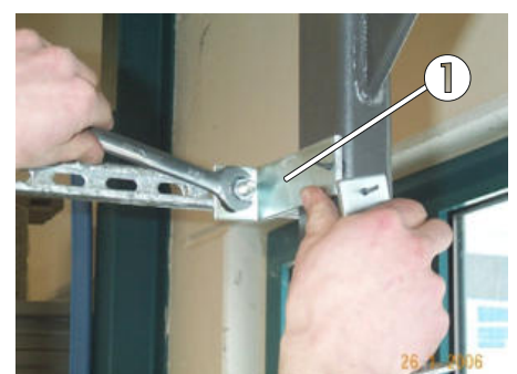
Fig. 44: L angle for the upper cross beam
