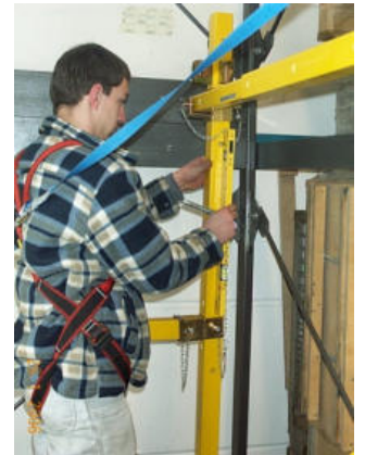
Fig. 60: Attachment of inner and outer tube with a short locking pin
