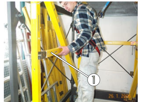
Fig. 63: Make sure you have the correct outer tube
