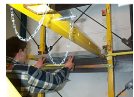
Fig. 85: Laying the upper floor panels
