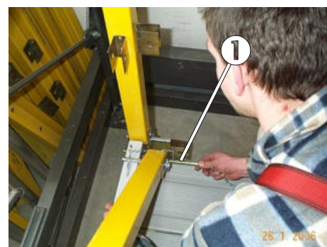
Fig. 66: Mounting the toeboards and midrails
