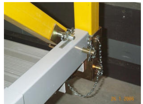
Fig. 68: Using a long locking pin to mount the rear, right-hand toeboard
