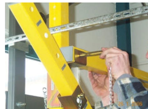
Fig. 58: Correct alignment of locking pins
