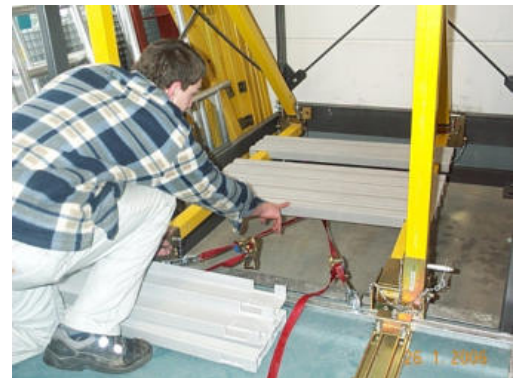
Fig. 32: Laying the other floor panels
