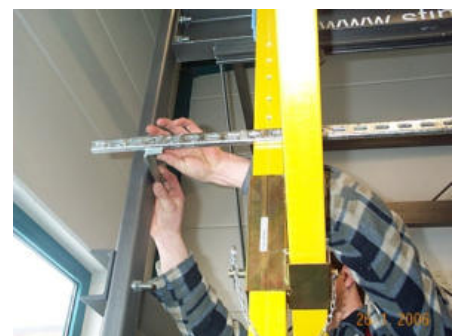
Fig. 43: Attaching the second L angle
