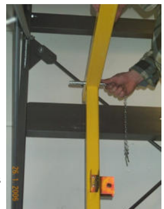
Fig. 94: The outer tube of the handrail is placed on top of the rear vertical rail stanchion
