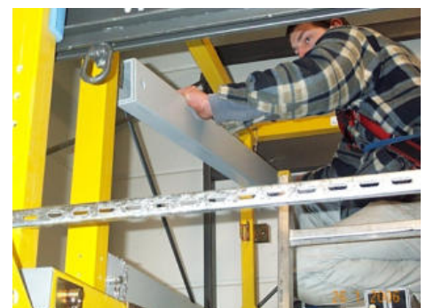
Fig. 98: Securing the toeboard
