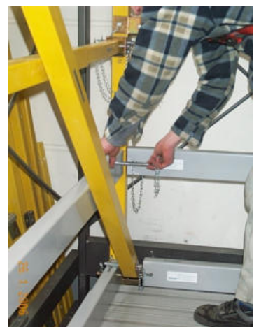
Fig. 72: Securing the midrail with a bolt
