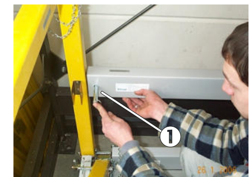
Fig. 70: Mounting the front midrail
