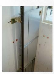
Details: Material steel plates made of galvanised steel 1.5mm
