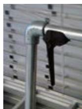
Linkage handle to extract the guard rail. Closed run of guard rail to avoid accidents
