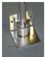
Safety switch to monitor the car guard rail position
