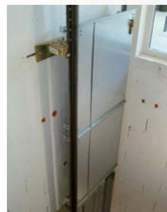
**Details:** Material steel plates made of galvanised steel 1.5mm
