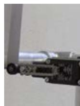
Safety switch to monitor the car guard rail position
