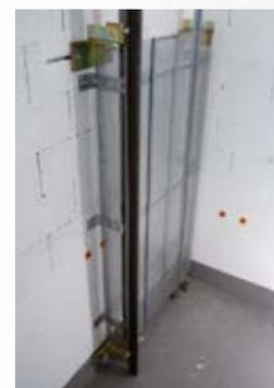
**Details:** Galvanised perforated steel plates (mesh width 8x8mm)
